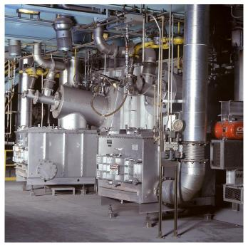
Figure 8 Pair of Regenerative Burners
